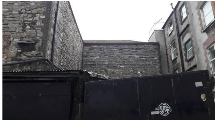
Side annex shed buildings
